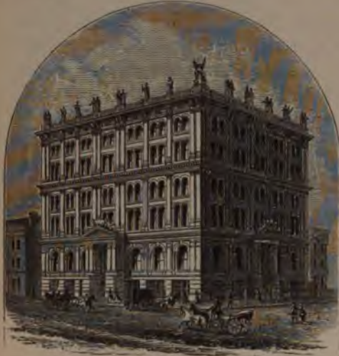
The St. Louis Life Insurance Company's Building.
